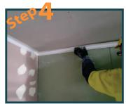
One person can easly put the PTT Ceiling Shadow Bead in place
