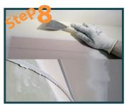
Special tearaway coming out leaving the shadow gap perfectly clean, just put a broad knife into the tearaway shadow where it fixed to the bead and it will pop out.
