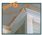
Miter Internal & external corners angles similar to the way you miter cornice corners
