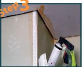
Lightly spray the ceiling & wall junction with the PTT Cornerbead Spray Adhesive, use the new PTT 42-EZYTRIG Spray Can Trigger to turn the can in a spray gun.
