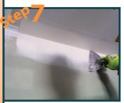
Setting is easier than setting an internal angle because of the special setting guides
